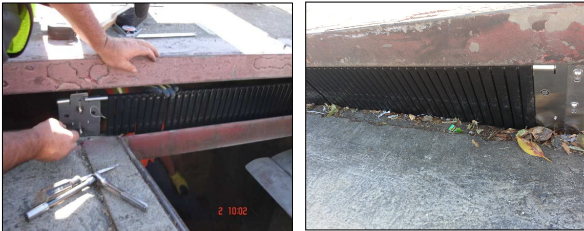
Figure 7. Curb Opening Screen Cover Shown in Open and Close Position
