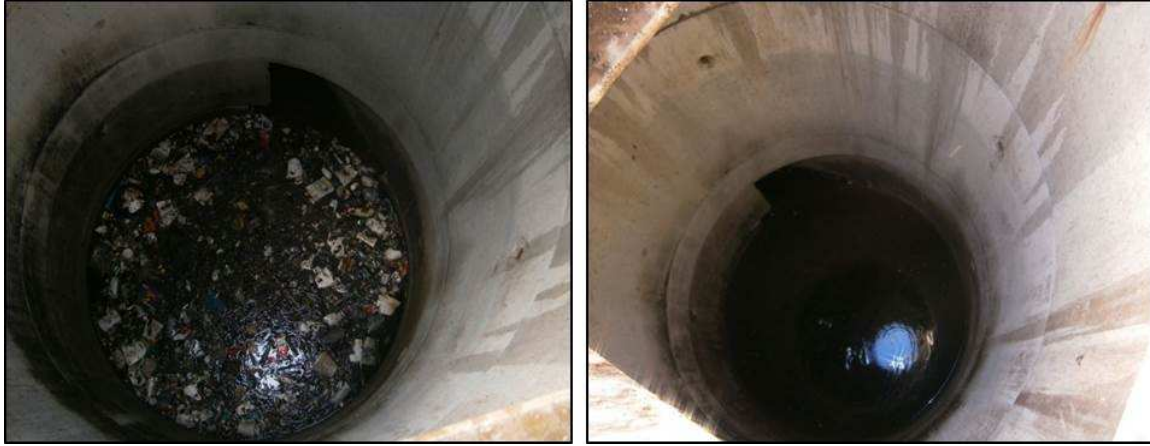
Figure 6. Photos Showing CDS Structure Before and After Cleaning
