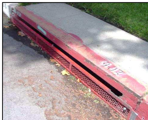
Figure 2. CB curb opening screen, fixed
